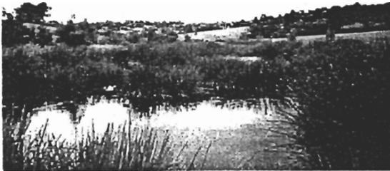
A constructed wetland system is a shallow waterbody system designed to regularly fill and drain. Wetlands tend to be heavily vegetated with emergent aquatic macrophytes which facilitate the removal of fine particulates and soluble pollutants. Wetlands are generally comprised of:
