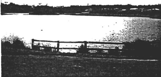
Ponds are open water bodies used as storage of stormwater runoff for reuse and/or to serve as an ornamental lake.
