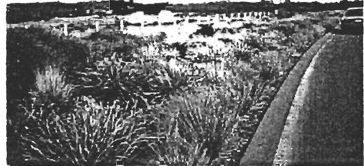
A grassed or vegetated channel can be used as an alternative to kerb and gutter or within POS reserves to convey stormwater runoff.
