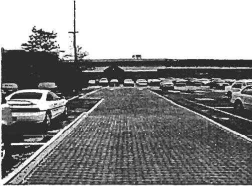
Porous pavements are an alternative to conventional road pavements. They consist of modular pavements cells with gaps between cells to allow infiltration of stormwater.
