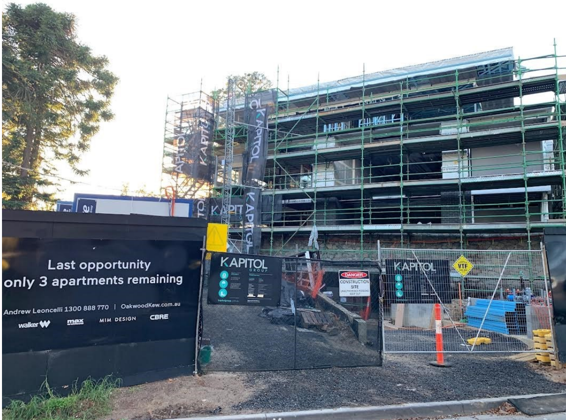
Kew Cottages Development, Stage 8 Apartments construction as at 23 May 2021
